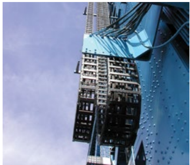
Nylatrac Modular TL carriers, with anodized aluminum crossbars for added strength in heavy wind conditions, maintain the lines for electric and hydraulic controls on a vertical lift bridge. Shown: The Main Street Bridge in Jacksonville, Florida.
