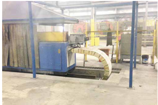
Enclosed-style Gortrac steel XL carrier in steel cable heat-treating application for unsupported long travel. Armor plates protect cables in aggressive environments.
