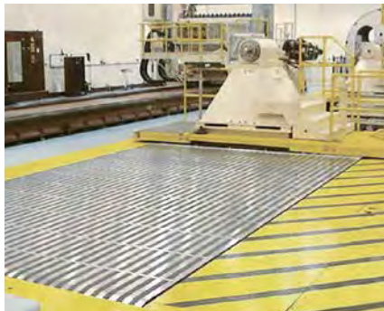
Machine pit with cover take-up mounted below the way
