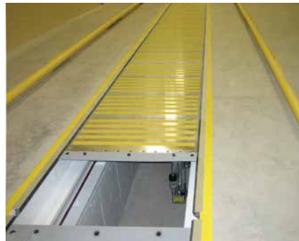
Vehicle inspection pit
