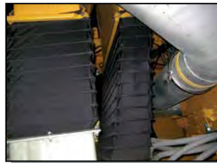
Air Ducting (exhaust, ventilation)
