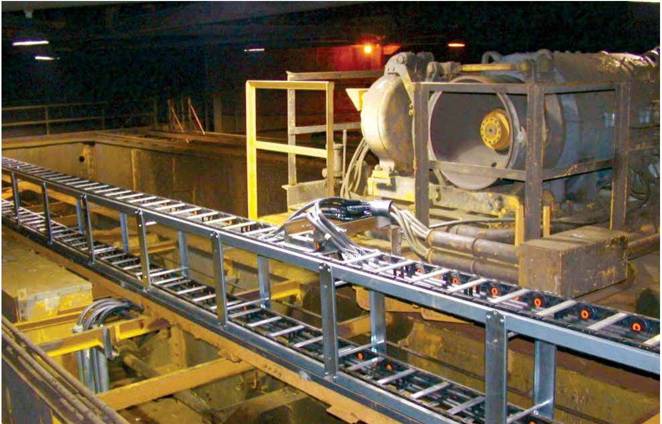
A complete cable carrier system designed by Dynatect includes a high-velocity rolling carriage and Nylatrac ® Modular TL carriers to achieve long travel in a steel mill.
